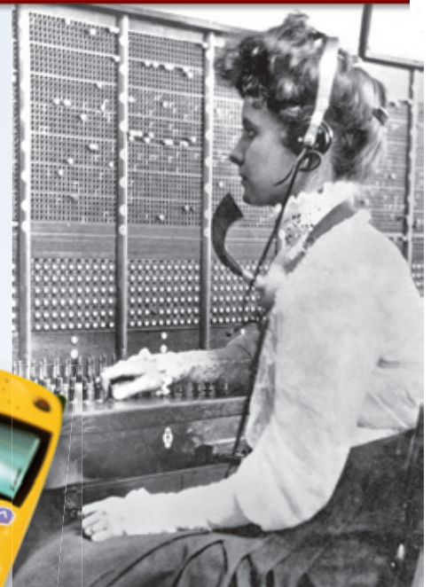
An operator connects two callers on a switchboard in about 1900.
